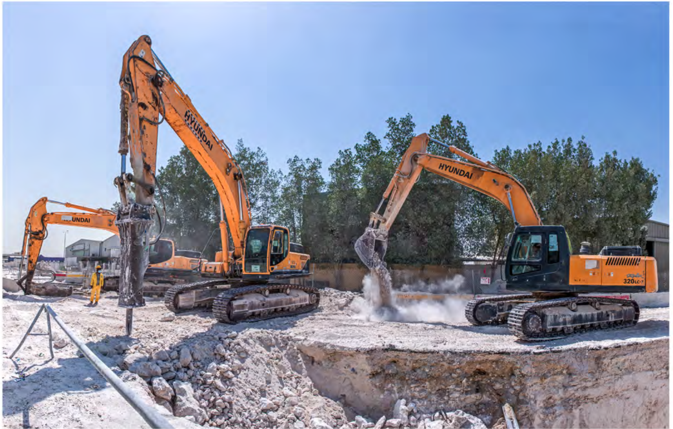
Road & Infrastructure in Doha Industrial Area Package 3
