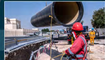
Construction of Diversion for foul Sewage from Doha West
