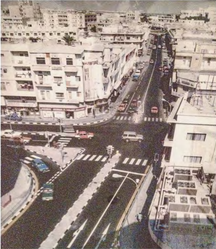
Abdullah Bin Thani Street Project; QBC Road Project was in Sofitel Junction, 1995
