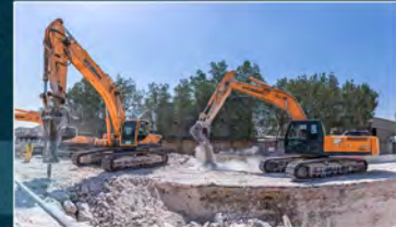
Road & Infrastructure in Doha Industrial Area Pck.3
