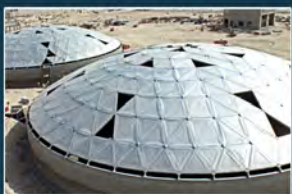
2016 Doha Port Infrastructure Roads & Utility Buildings
