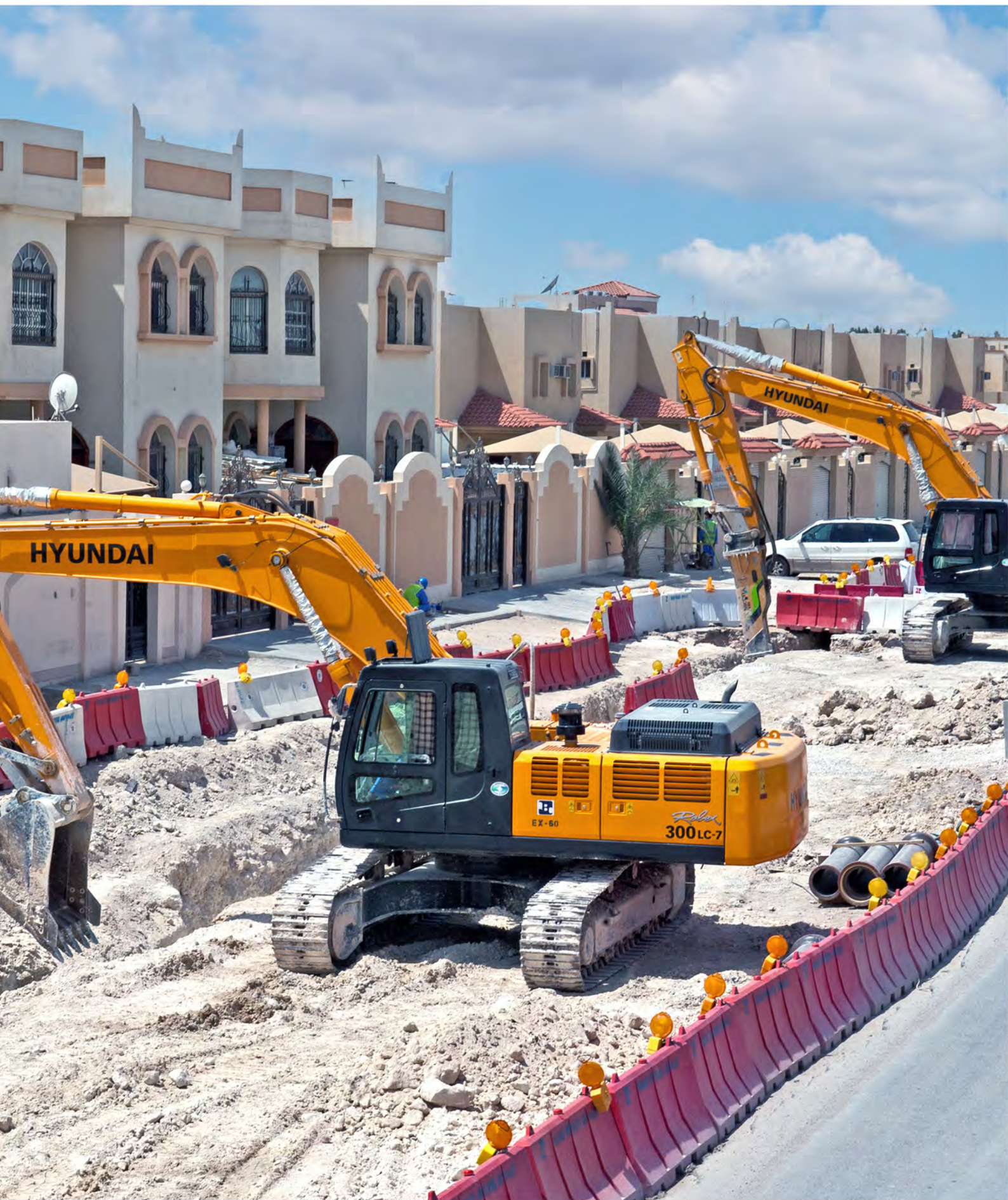
Construction of Al Nassriya Area Sewerage Phase3 / CP 745
