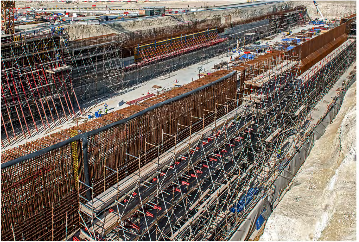
Reinforcement & Scaffolding work for the underpass at CP07A-1A Waterfront Commercial/Seef Lusail South Infrastructure Project
