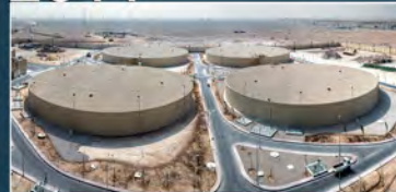
GTC 299 Al Wukair RPS & Associated Pipelines
