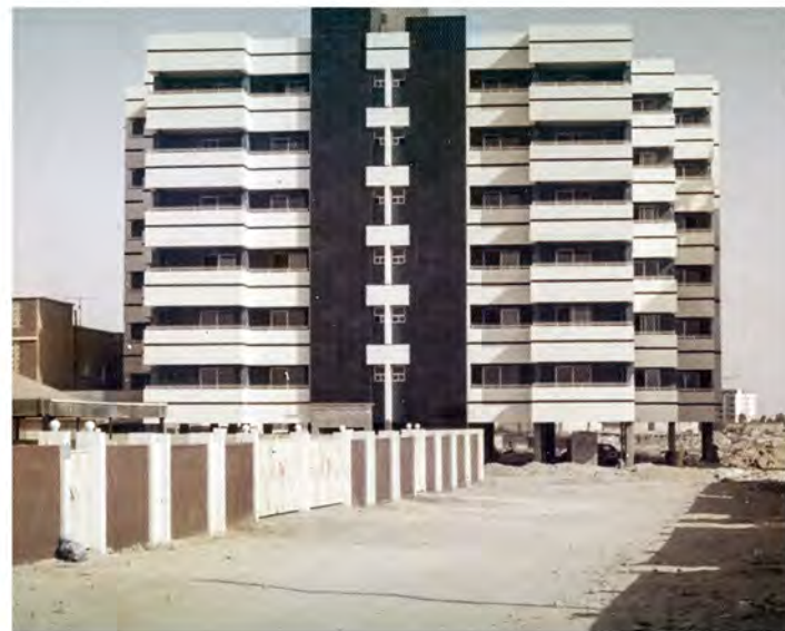
The first multistorey building project was a Residential Building in 1975
