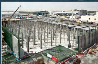
GTC 269 New Reservoirs & Associated Pipelines at Gharrafa
