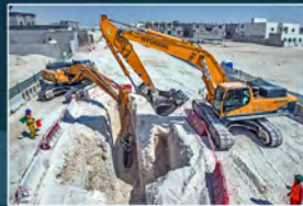
2015 Roads & Infrastructure in Al Sailiya North of Salwa Road
